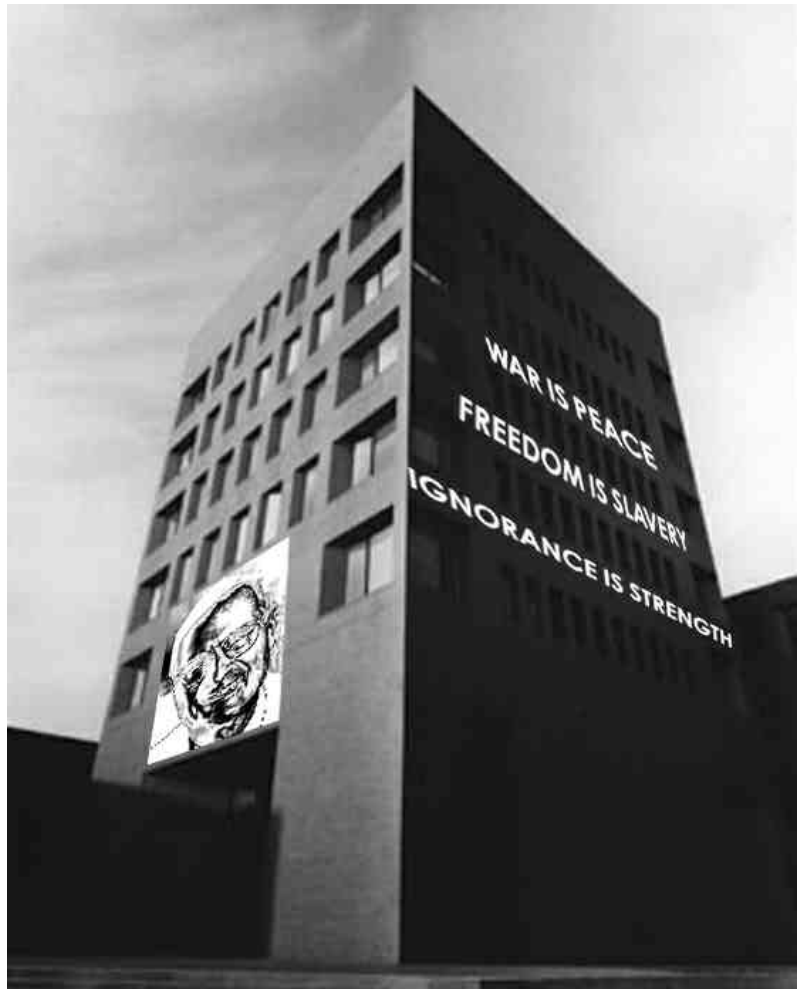
The Frank Lamas Building, Building #1984
